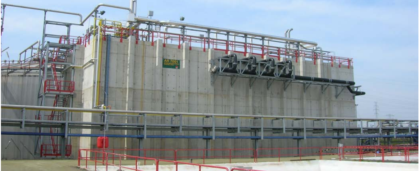
BP Geel New Waste Water Treatment Bioreactor Geel, Belgium
