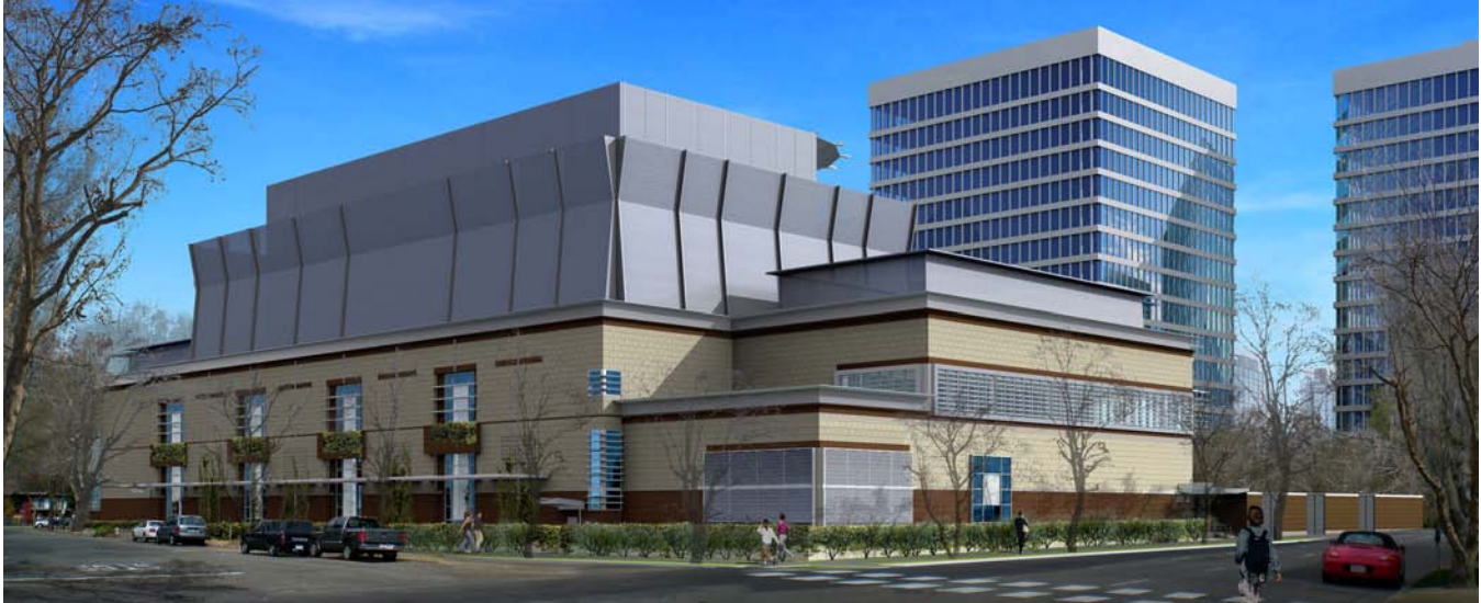
Department of General Services, State of California Central Plant Renovation Sacramento, California
