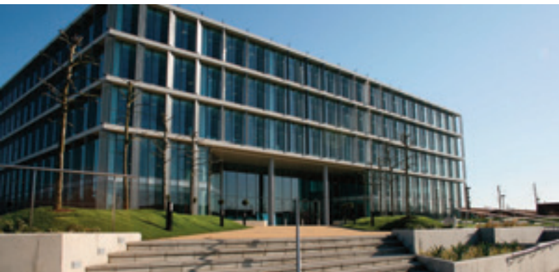
Manchester office, England, United Kingdom
