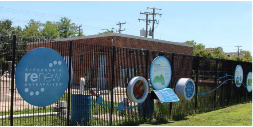
Interactive Educational Exhibits at AlexRenew's Four Mile Run Pump Station
