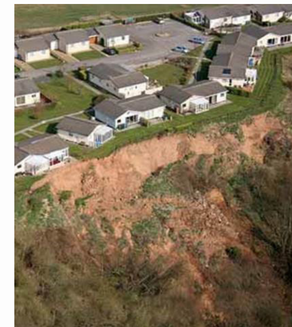
Figures 6.17. & 6.18 (left): Coastal landslide impact on residential properties at Knipe Point. Images courtesy: Moore (bottom left); Scarborough Borough Council (bottom right).
