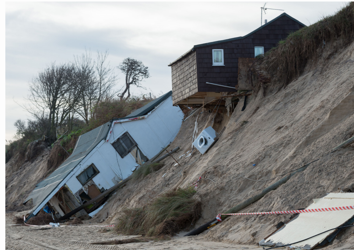
Figure 3.4 Damage to coastal properties caused by the tidal surge and flooding on 6th December 2013 at Hemsby, Norfolk, UK. Small coastal communities along undefended coastlines are particularly vulnerable to the impacts of cliff instability, erosion and climate change Image courtesy: Alamy Stock Photo/Jon Gibbs.
