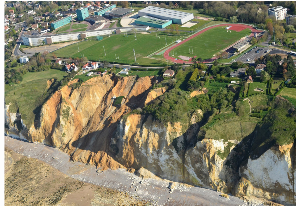
Figure 6.27 Shows the landslide in December 2012. This led to a failure of over 100,000 cubic metres of sands and clay and cliff retreat of over 40 metres. Since then landslide activity has continued. Coastal residences at risk were purchased with funds provided through the provisions of the Barnier Law.
