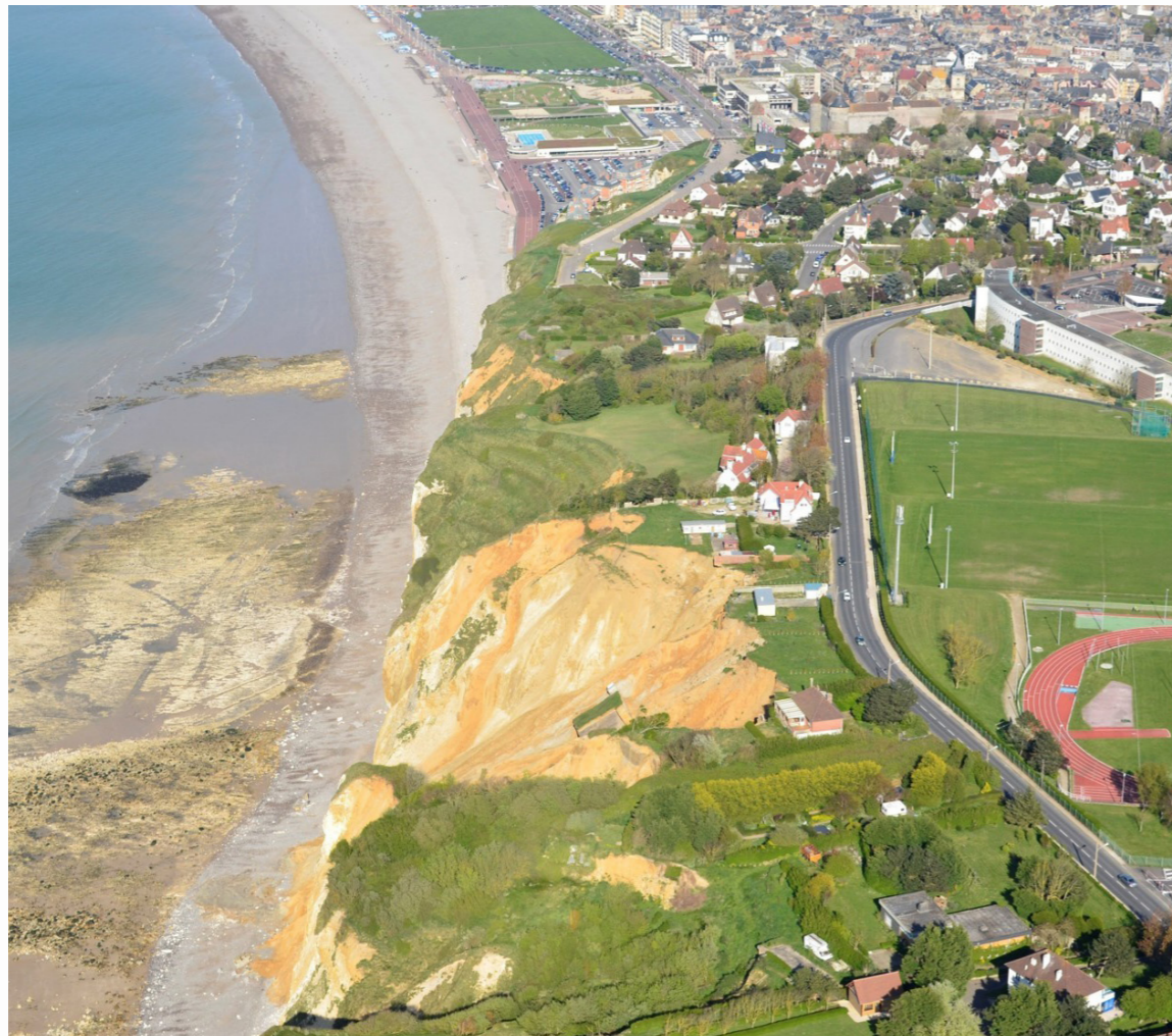
Figure 6.26 View of the cliff failure looking north-east towards Dieppe. Image courtesy: © Thomas Dewez, BRGM.
